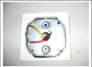
Using a razor knife, remove all the paper inside the  $4 \frac{1}{4}$ " x  $4 \frac{1}{4}$ " square. You will also need to remove about 1/8" of sheetrock so that the plate on the back of the sconce is recessed. This will allow the sconce to lay flat against the wall.
