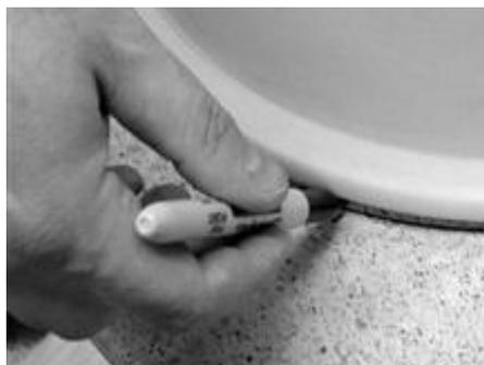
**7. Apply a 1/2" bead of 100% silicone sealant to the top.**
