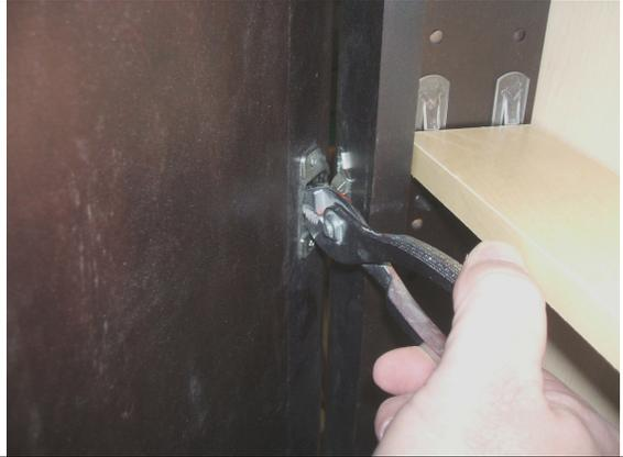
4. Slowly close door allowing the nose of the pliers to be closed up in the hinge until you hear a slight pop or creaking noise as shown in picture
