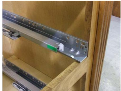
3. Place one or more shims with the lip of the shim inside the cabinet and the screw hole centered in the slit of the shim.
