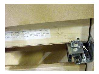
The soft close drawer glides have an adjustment on the back of each glide that can help adjust the vertical alignment of the drawer front. Move the lever (shown above) left or right to adjust. This will raise or lower the back of the drawer box.
