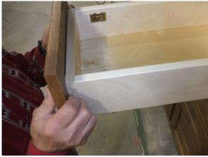
Pull the drawer front out to the end of the glide. Push drawer to the right to adjust to left side. Push the drawer to the left to adjust to right side.
