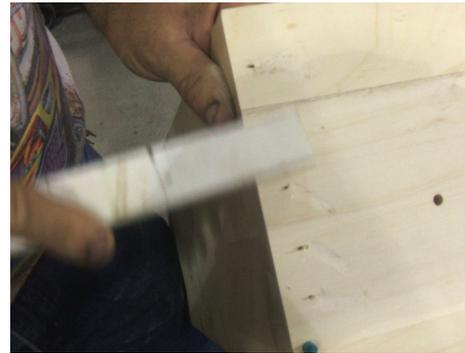
9. Measure the distance between the bottom of the hole and the bottom edge of both replacement and original drawer front to ensure proper drilling.
