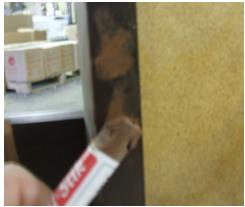
4. Remove any excess filler and level the repair using a plastic card.
