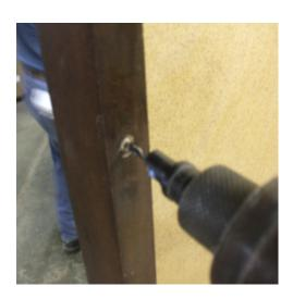
5. Replace screws. If your drill has a torque adjustment (clutch), turn the torque down to avoid stripping the repaired holes.
